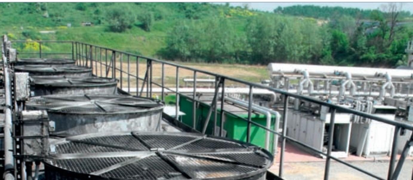
*Fans provide steam cooling, turning it into water*
